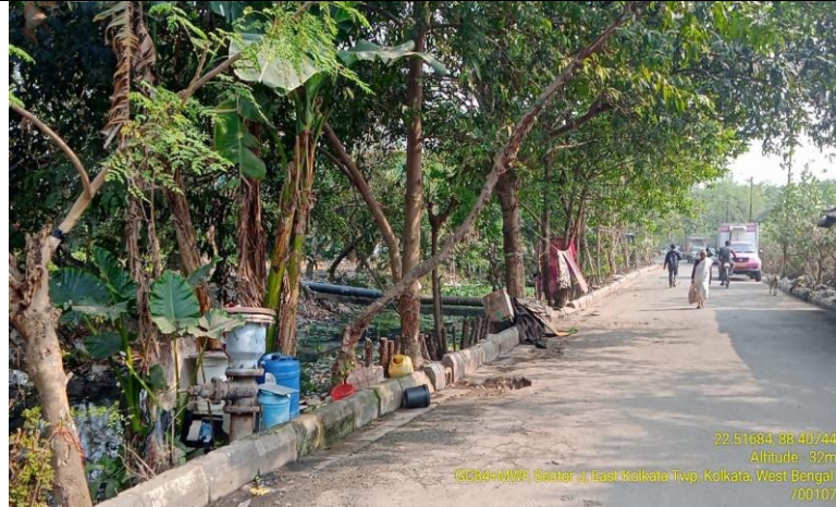
Outfall near Sanchi International
